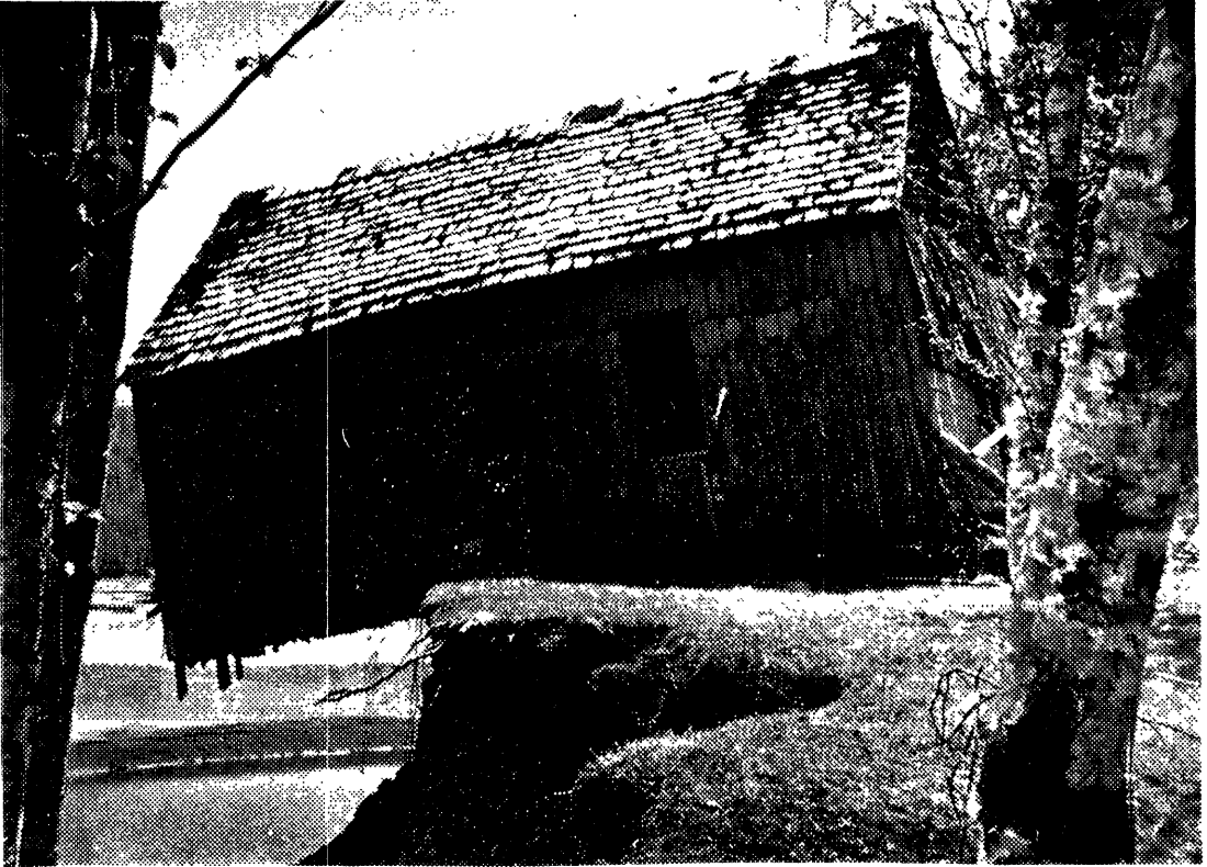
In The River Now—This is a scene of the home of the William Moritz Homestead located down stream from Westward Hoh Resort on the Hoh River. The unit was built in the 1890's and in about 1916 the river was about a mile away from this building. This photo was taken May 5, 1968 and since that time the unit has slid into the river. Moritz attempted to have a hops farm at this location.
